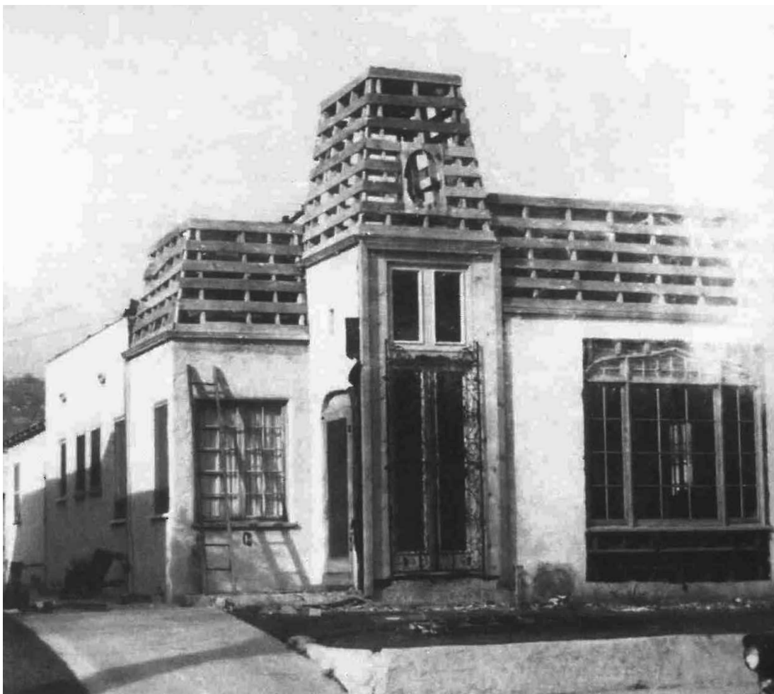
Roof framing complete at the Limotti-Worsley house. Photo by Larry Limotti.
