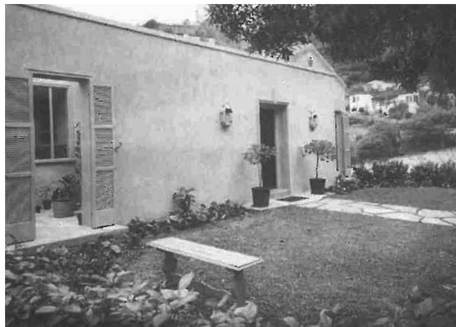
8488 Carlton Way, West Hollywood Hills, c. 1946. The remodeled Frank L. Anderson house. It is the first published West Hollywood remodel that uses a screen wall placed in front of the street facade for added privacy. Photo by Maynard Parker.
